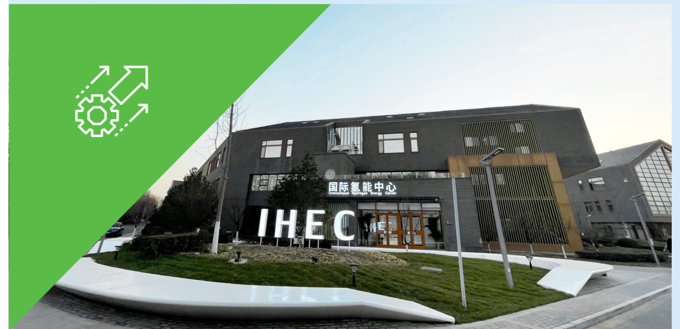
International Hydrogen Energy Centre located in Beijing, China.
