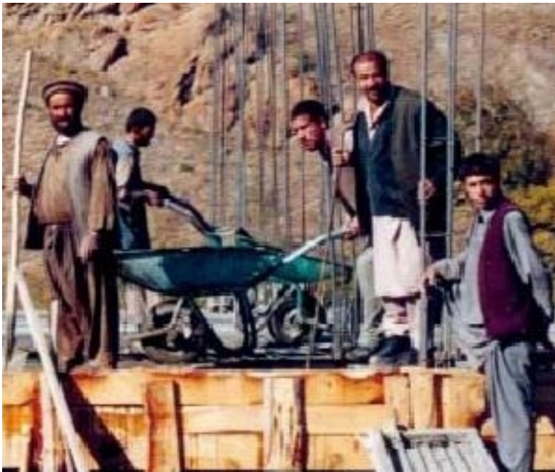
A construction site in Afghanistan
