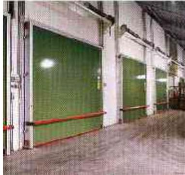
Doors may be mounted on a sliding rail, as pictured to the left. Or, they may be mounted to open vertically on overhead rails, as pictured to the right.
