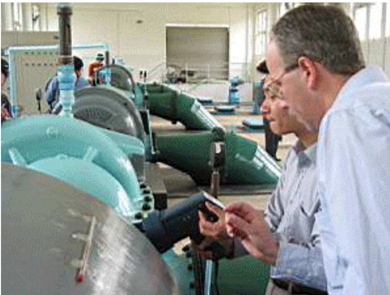
Improving the efficiency of motor systems raises productivity and lowers pollution
