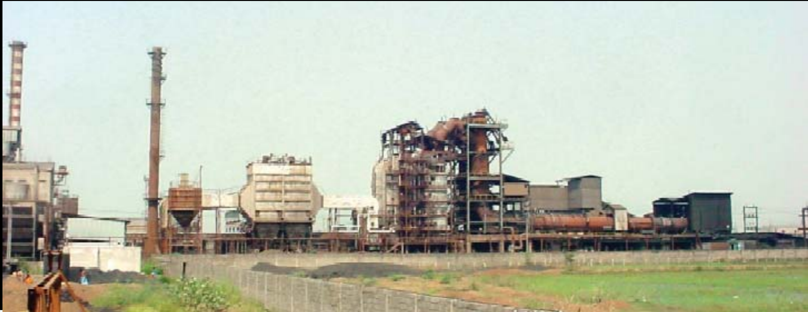
8 MW Waste Heat Recovery Captive Power Plant, Raipur, Chhattisgarh
