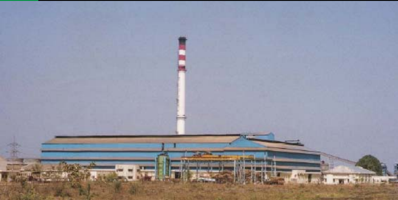
22 MW Cogeneration Project, Nagpur District, Maharashtra
