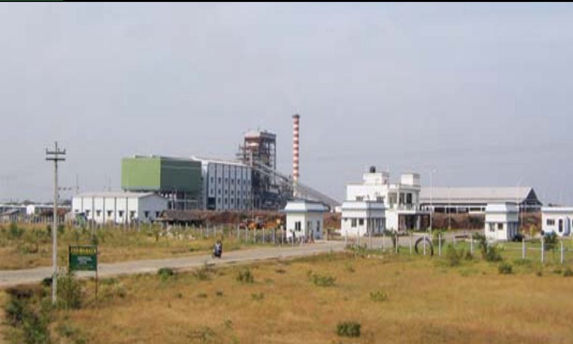
20 MW Biomass Power Project Turicorin District, Tamil Nadu
