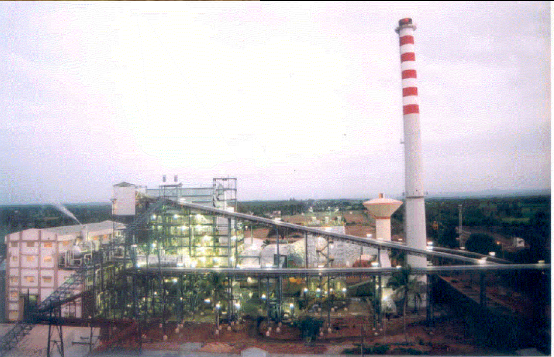
24 MW Baggase Cogeneration Power Project, Davengere District, Karnataka
