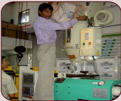
Material feeding system in hopper
