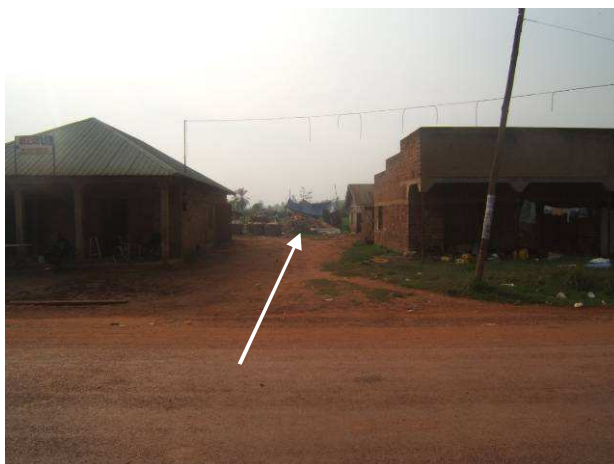
Figure 15: A side View of Bwaise Plastic Recycling Plant
