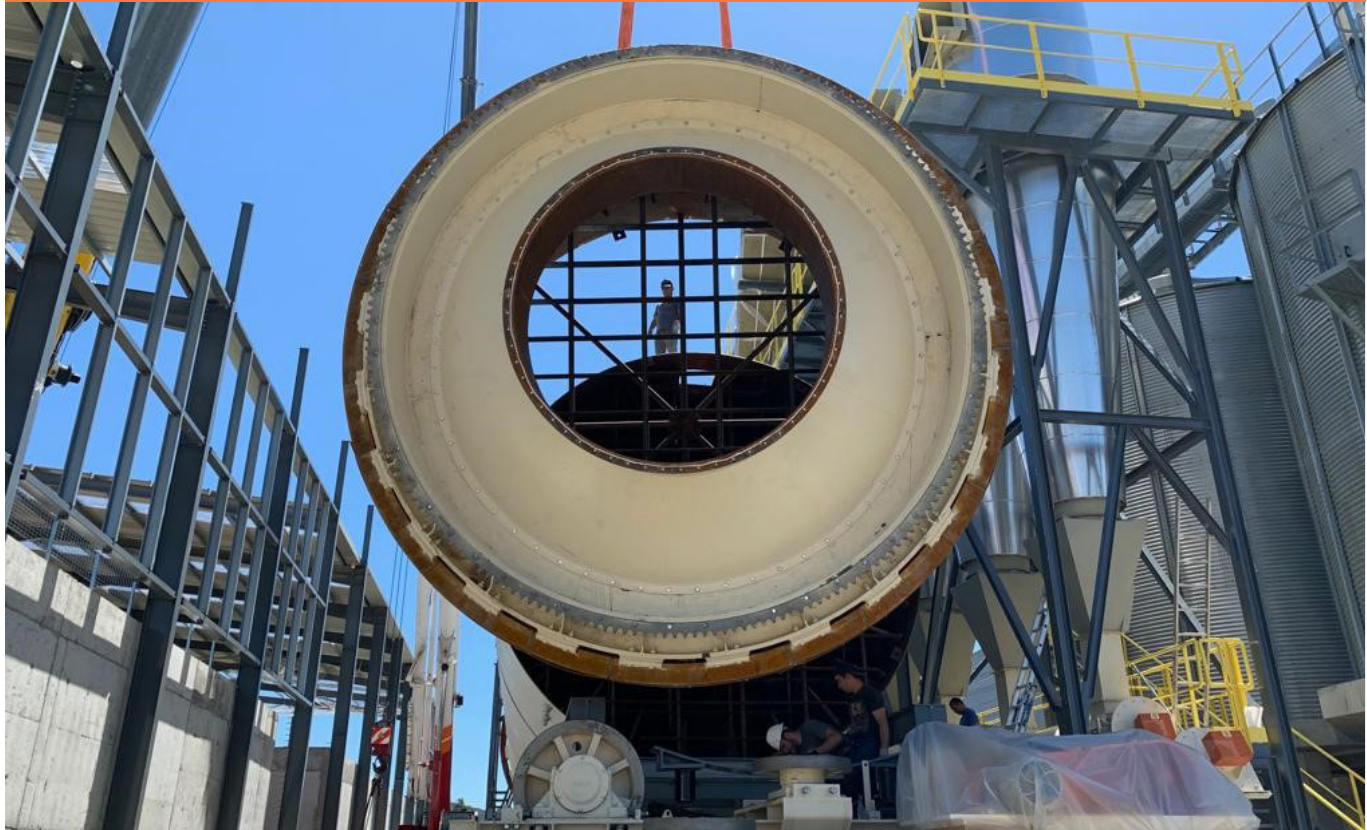
Installation of drying/torrefaction unit. (Source: Futerra Fuels)
