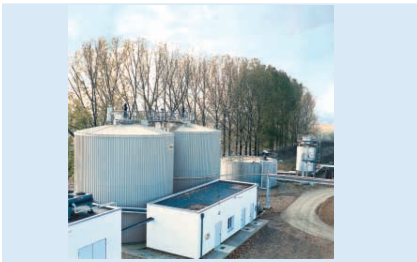
Figure 6: General view of the Behringen co-fermentation plant in Germany
