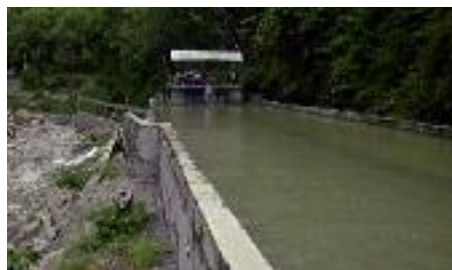
Figure X. De-silting tank
