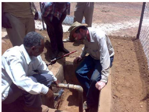
Fig. 3: Laying pipes and utilities for water to set the foundation for the Wau VTC to become a functioning learning centre
