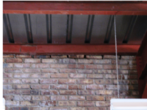
Mortar washed out from brickwork at wall plate level
