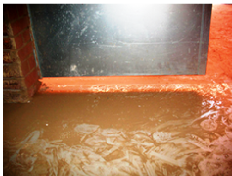
Large (4cm+) gaps at bottoms and tops of exit doors
