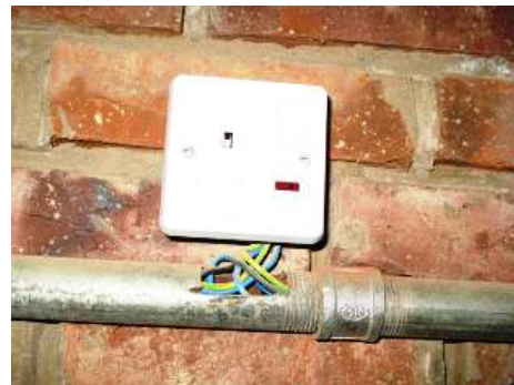
Sharp pipe edges not filed smooth, screws in low quality mortar
