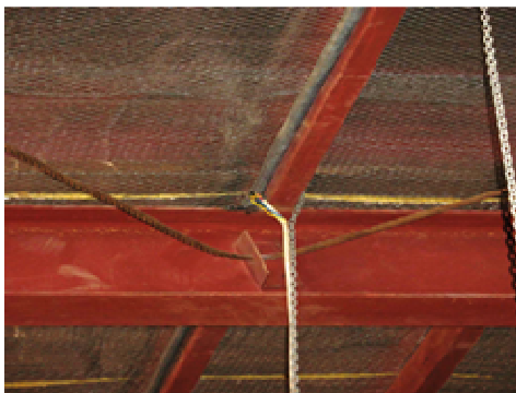
Cables designed to tension the building steel frame are already slack in places
