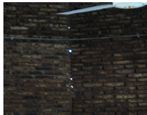
Daylight seen through the corner of a workshop
