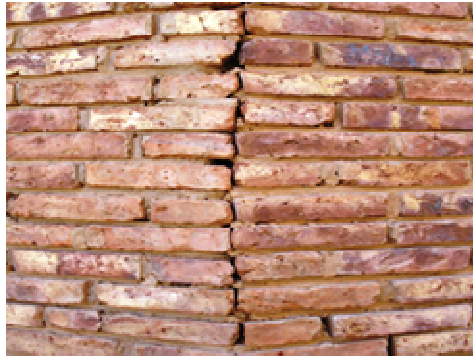
Corner brickworks not interleaved
