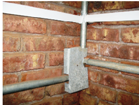
Method of bonding conduit and covering joint
