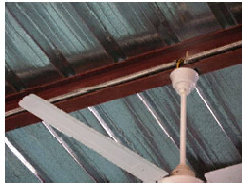
Ceiling Fan Connection
