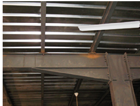
Roof support joists do not rest on structural steel – attempt made to weld them in place
