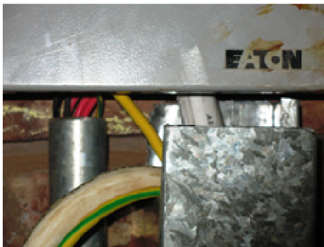
Connections to Main Distribution Board
