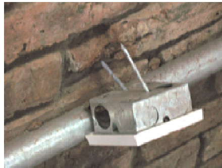
Smooth nails into poor quality mortar to fix box
