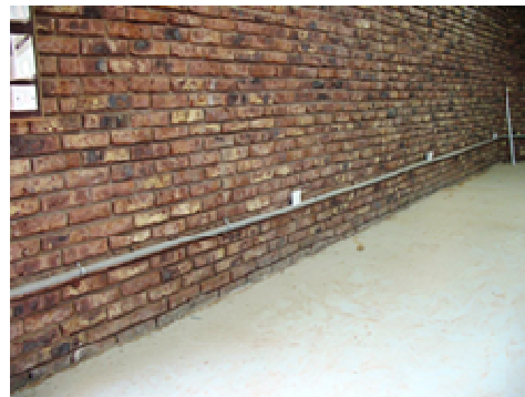
Walls poorly pointed. Would be better plaster or concrete skin finish and painted white to reflect the small amount of available daylight
