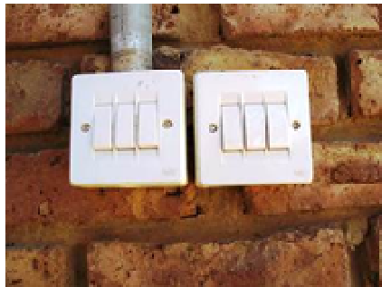
Internal type switches fitted on external wall – NOT WATERPROOF
