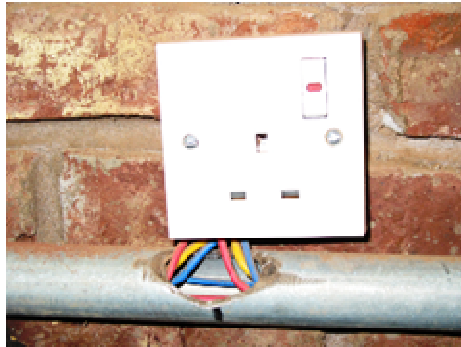
Typical Single phase power socket installation
