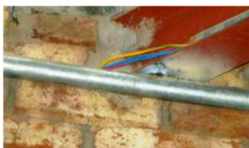
Figure 1. The figure shows how the wires connection go from one wiring pipe to the other one, without any protection. The yellow, blue and red wires are not double insulated and are in any case supposed to run inside a pipe. The pipes are not connected to any reliable earth terminal. Every single piece of pipe should have its own connection, while the connection between each piece should be properly carried out and tested.
