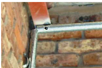
Figure 2. The figure shows the angle connection with interrupted pipes, i.e. without a curved joint that guarantees the continuity of the pipe itself.
