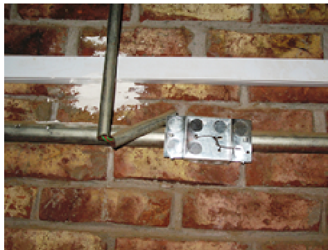
Method of bonding conduit and covering joint
