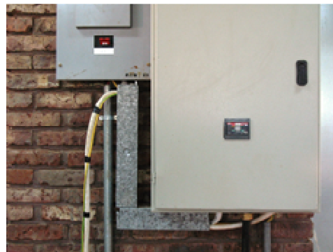
Connections to Main Distribution Board
