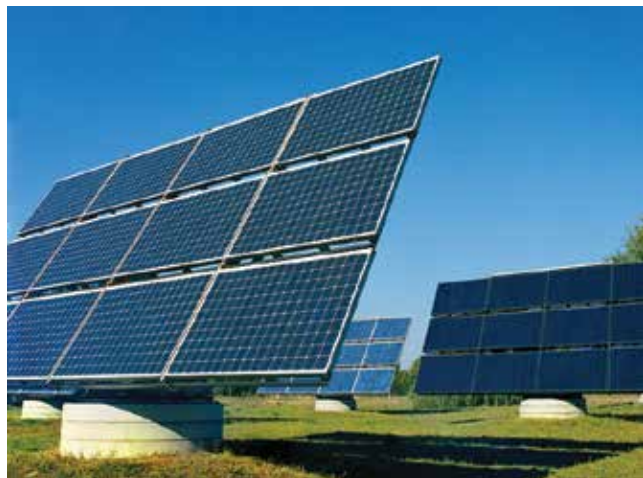
Figure 9: Use of Solar Energy in MSME industrial sector
