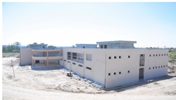
Construction complete at the Yirgalem IAIP (SNNP region).
