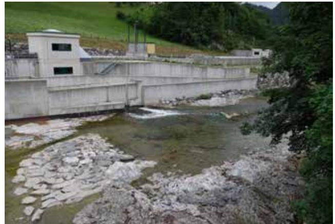
**Figure 3.** Fish pass and residual turbine at the Opponitz hydropower plant
