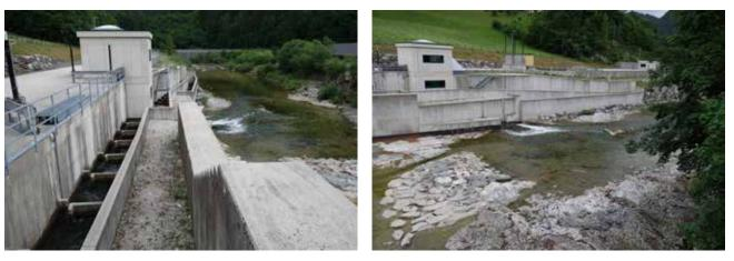
Figure 3. Fish pass and residual turbine at the Opponitz hydropower plant
