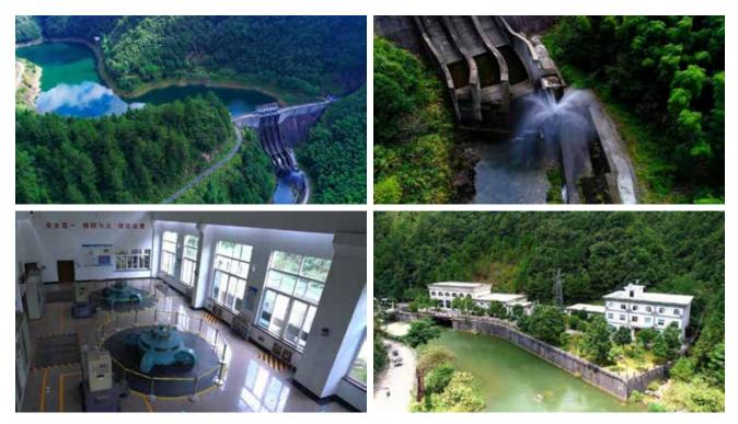
**Figure 5.** Anming First Cascade in Songyang, Zhejiang Province Note: Total capacity is 2 x 6.3 MW, reservoir storage capacity is 3.32 million m3, an 80 cm pipe was installed at the bottom of the reservoir for ecological flow discharge.
