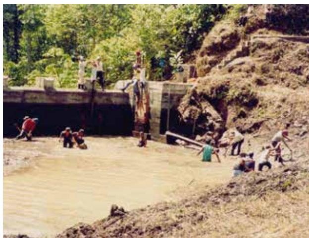
Figure 6. Annual cleaning of sediment from the headpond at Bocay
