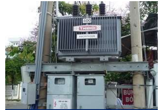
High efficiency transformers in power grids (Viet Nam) 7,972 tCO 2 /y. Start operation 2016-2018
