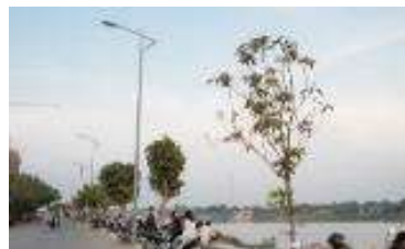
LED street lighting system with wireless network control, MinebeaMitsumi, Cambodia
