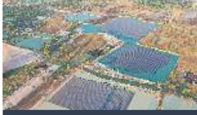
Floating Solar PV, TSB Co., Ltd., Thailand
