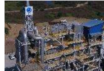
Waste to Energy Plant, JFE engineering, Myanmar
