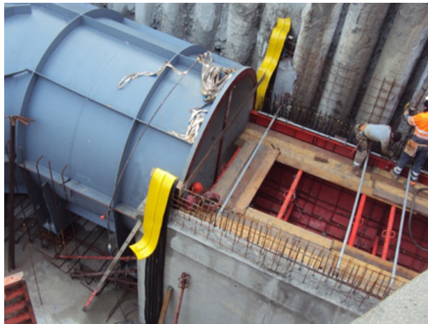
(g) second phase of concrete casting
