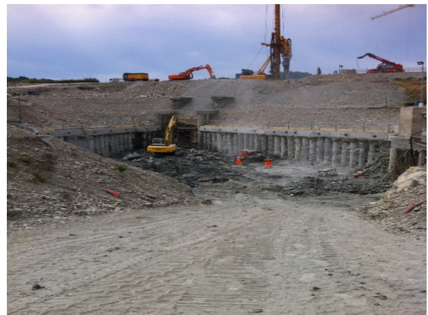
Figure 4. Working phases: (a) building of secant poles
