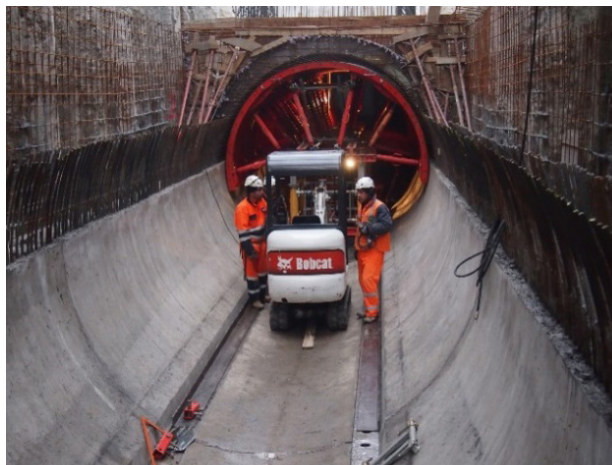
(g) second phase of concrete casting
