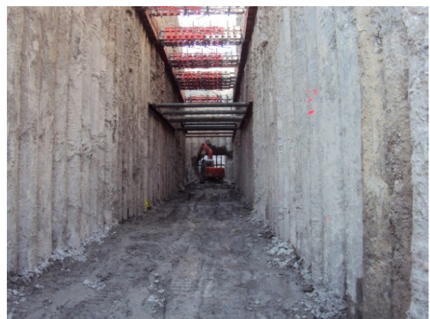
(b) support and excavation
