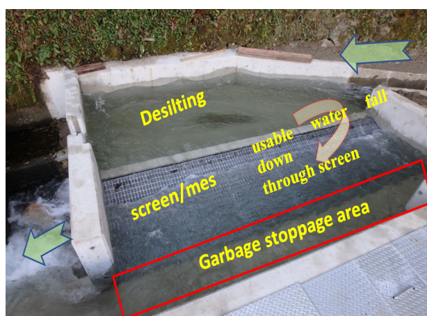
Figure 3. Forebay tank and desilting tank
