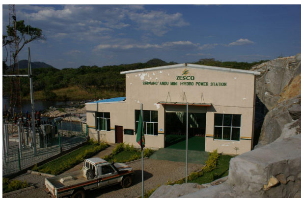
Figure 3. Shiwang’andu SHP plant
